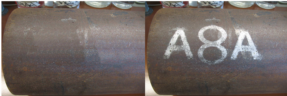
III. 1: Rusty stovepipe
